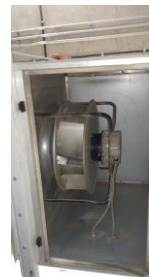
EC fans for AHUs, UFADs, Exhausts, DOAs
